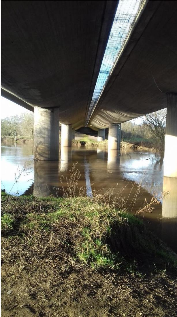
This is a strange unremarkable photo, viz the underside view of the bridge over the A64. However, it indicates that the structure is virtually 2 bridges. The gap between the 2 sets of dual carriage way is merely filled in with a wire mesh.
