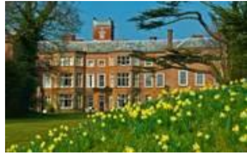
Claydon House surrounded by spring bulbs.
