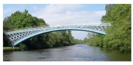
Meandering on upstream, we see the Aldford Iron Bridge. We sail under the bridge and turn round. Built in 1800's by a Chester Victorian Architect, John Douglas and completed in 1824 by William Hazeldine for the first Duke of Westminster. Bridge span is 150ft and a roadway width of 16ft. The bridge of course was inspired by Telford's Iron Bridge over the River Severn in Shropshire.
