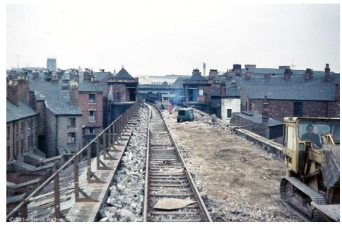
Arkwright Street station (being demolished, the platforms already removed).
