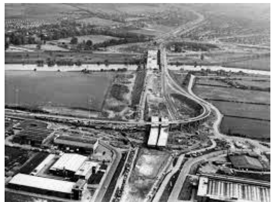
...and the second bridge and flyovers under construction 1972....
