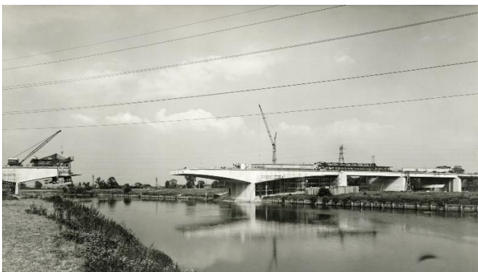
First bridge under construction 1957....
