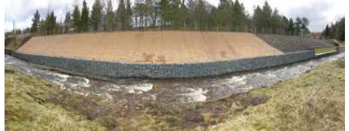
Nenthead car park river bank completed © Environment Agency
