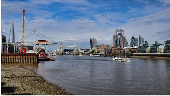
Chambers Wharf Jetty Tower Bridge & City
