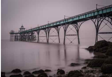
Clevedon Pier, Britain's only Grade 1-listed pier
