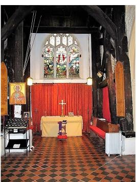
The nave is early 13th century with the roof replaced in the 15th century and is of the braced collar-beam type with two king-post trusses.
