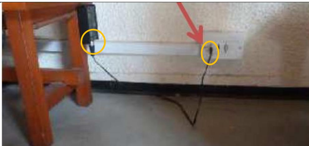
There is a large to small diameter conversion plug left in the top of the junction box. Remove that and place it on the window ledge above. And fit the U3A larger diameter plug into the top of the junction box.
