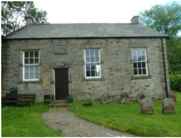
The Friends Meeting House over the river and on the left of the road, founded in 1735
