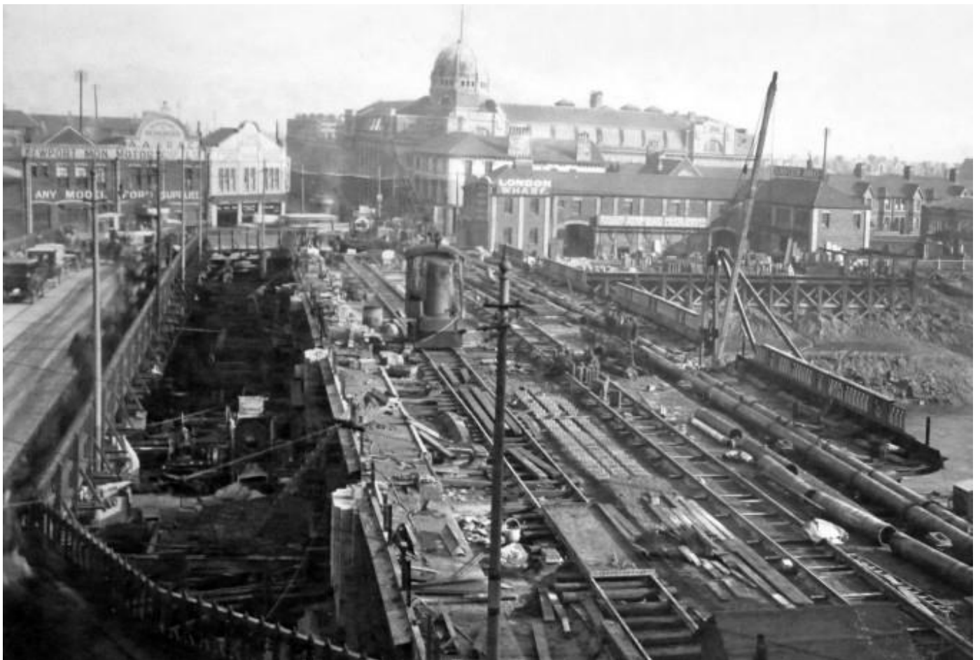
Rebuilding of Newport Bridge, 1927 Temporary bridge to the left of the new structure
