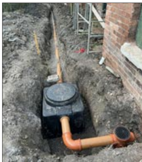
New pipework installed
