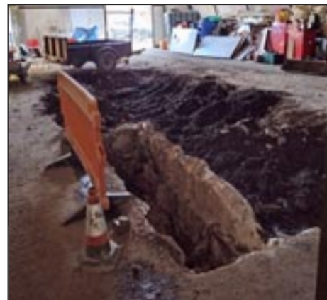
Digging up the floor of the Romney building
