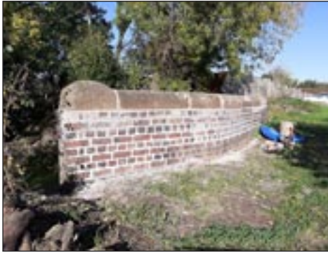
Widows Bridge repointed
