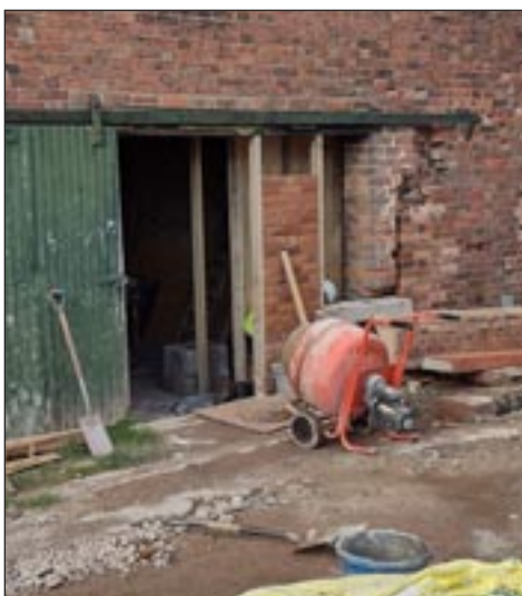
The new doorway taking shape
