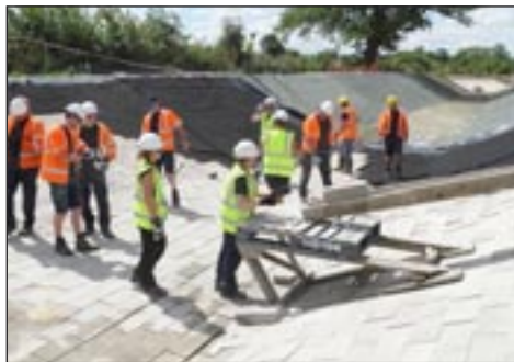
The block laying team.
