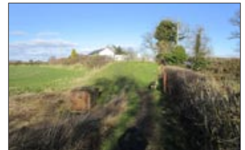
View from the towpath towards Schoolhouse Lane. The road is high above the canal, but it needs to be even higher for the canal to go under it
