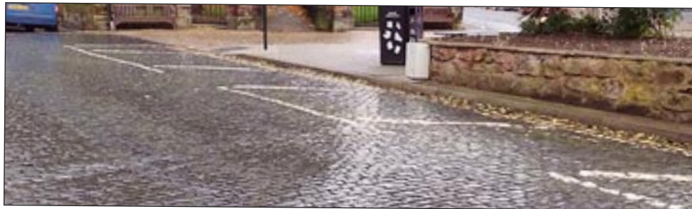
Granite Setts on St Mary's Street, Newport
