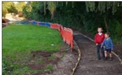
The new footpath and drain are installed
