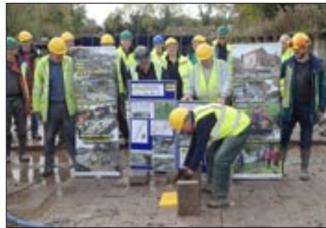
Laying the final block
