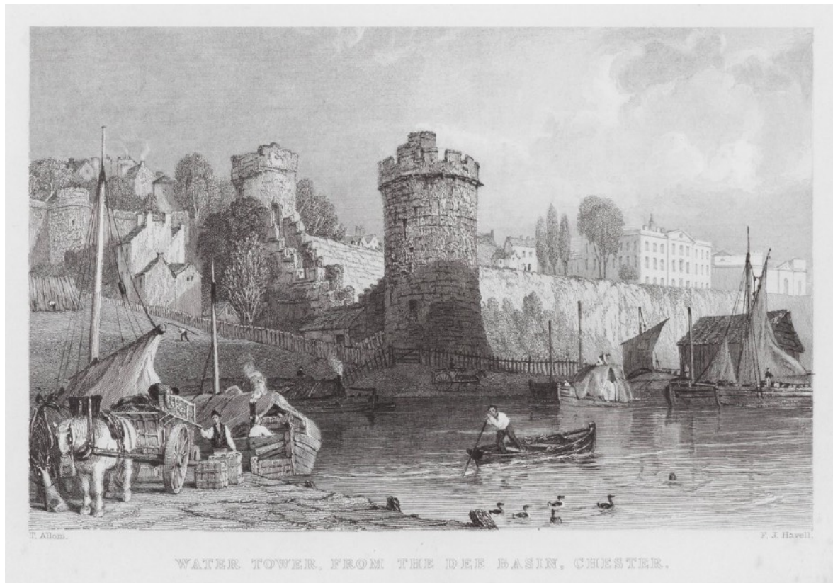
The Water Tower, from the Dee Basin, Chester (engraving) by Thomas (after) Allom
