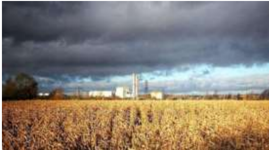
Staythorpe Power Station
