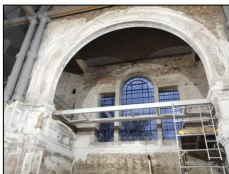
One of the church's restored windows
