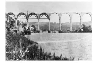
Calstock is dominated by the magnificent railway viaduct which was built between 1904 and 1907 by John Lang of Liskeard. Constructed from 11,148 concrete blocks it is the largest viaduct to built in such a way in Britain.
