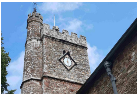
The one handed clock on the tower
