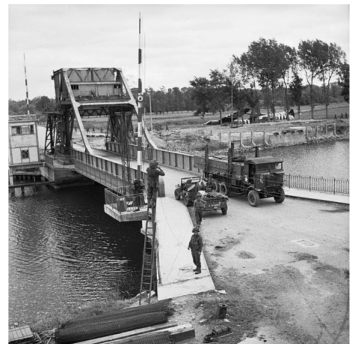
Caen Canal Bridge
