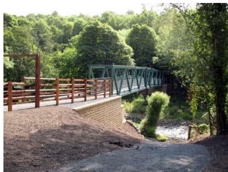
The current bridge.
