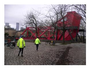
The original Bascule design (for example, Tower Bridge) used a single large axle, whereas the rolling lift bridge has a weighted counterbalance that rolls back on a hinge. There is a video of the bridge opening at: <u>https://www.mfoot.com/blog/2016/06/26/historic-remnants-1-the-bascule-bridges-of-rotherhithe-and-surrey-quays/</u>
