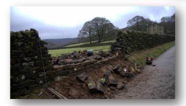
Once the footings are in we begin to put the first courses in. This was a difficult wall because there is a bank from the base to the road, and most of the stone had collapsed on the field side, probably due to earth movement over the years.
