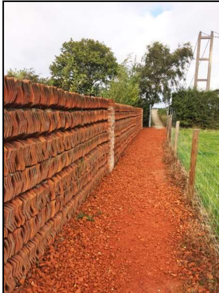
Walls made from terracotta roof tiles!
