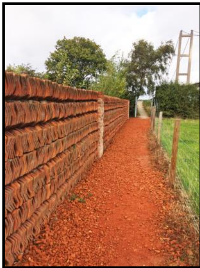
Walls made from terracotta roof tiles!
