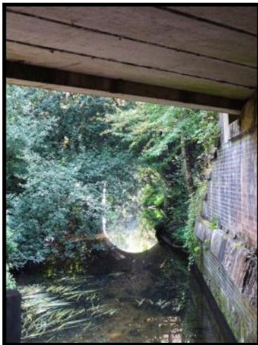
Rail bridge over Mother Drain
