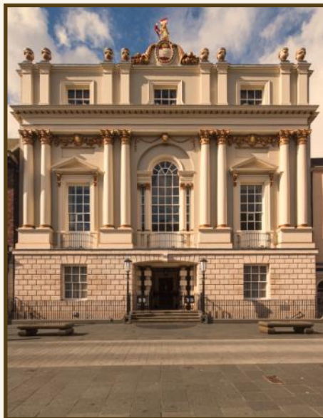
Doncaster Mansion House
