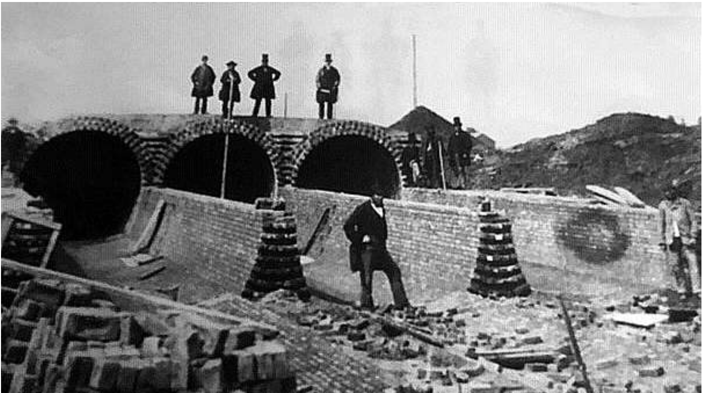
Mills pumping station, Stratford, London, in 1862.
