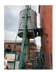
and locks. There are now three electric pumps in the adjacent room. We saw a demonstrate of how it all worked. In the adjacent tower a 100 ton weight is lifted up above a tank. The weight then slowly falls to pressurise the water in the hydraulic pipes. This accumulator ensures a smooth delivery of pressure, including peak demand, without needing to run the pumps continuously. We visited the maintenance workshops, also from the 1880s. Much of the original machinery survives.
