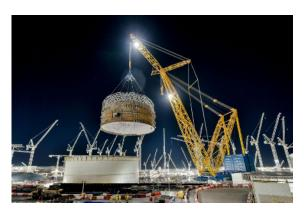
The tour continued past the jetty, where large items arrive by sea, several concrete making plants, and on past the first of the two reactor pressure vessels. Each ring of the vessel is assembled on site before being lifted into place by 'Big Carl', the world's largest crane.
