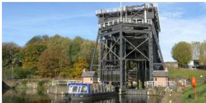
This massive iron framework lifts canal boats 50ft from the River Weaver up to the Trent and Mersey canal.
