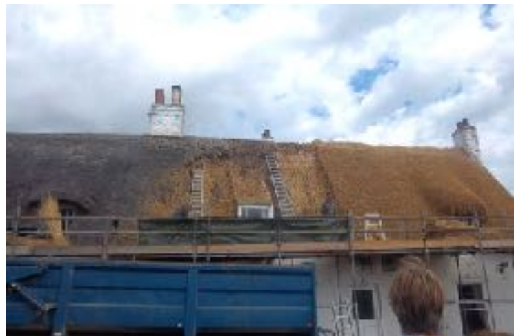
The New Roof at Ailby
