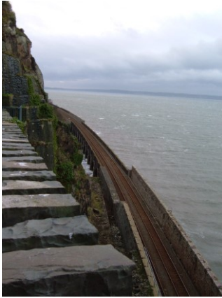
Railway on masonry arches alongside old Pen-y-Clip Tunnel route.
