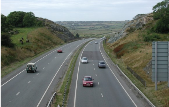
Near Pentre Berw the bedrock changes to hornblende schists which are more resistant to erosion, forming a prominent ridge. This ridge required a 17m deep blasted rock cutting.
