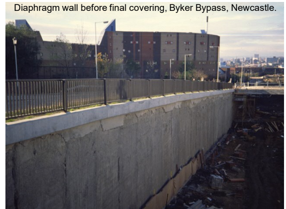
Diaphragm wall before final covering, Byker Bypass, Newcastle.
