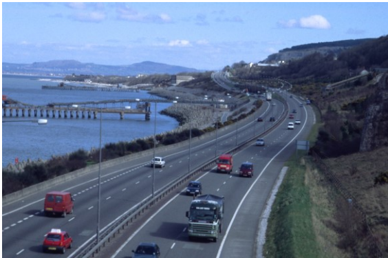
Just East of Old Colwyn – old complex landslips in glacial till over limestone.
