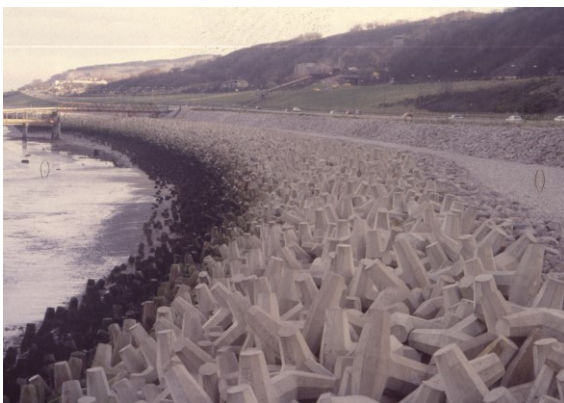
Constructed toe weight embankment needs marine erosion protection
