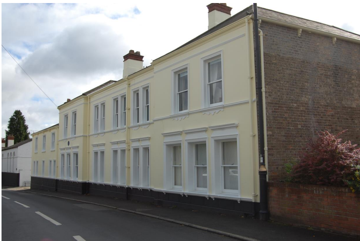
‘The Old Hall’, No 10 Church Lane, 2017
