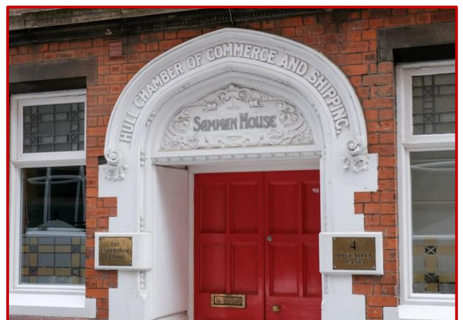
Samman House, Bowlalley Lane, Hull
