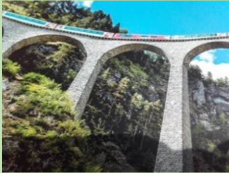
Landwasser Viaduct, Switzerland
