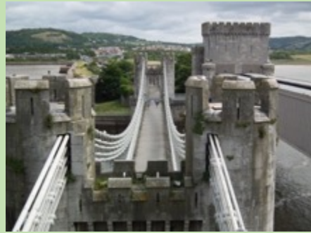
Conwy Suspension Bridge
